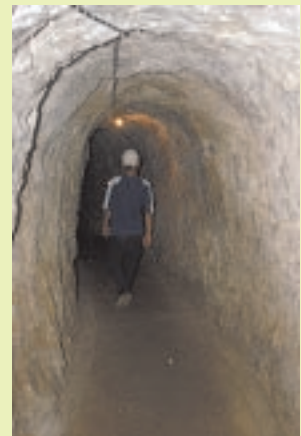
Pathet Lao tunnels were hewn using primitive tools.
